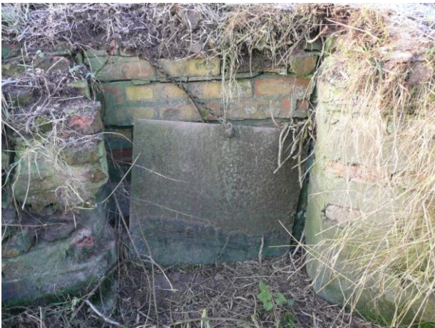
Fig 7 Photo showing the old flood-gate
