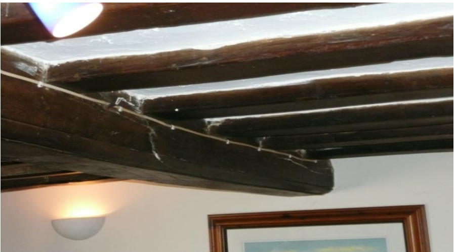
Figure 1. Beams in Number 21 Castle Rising.
